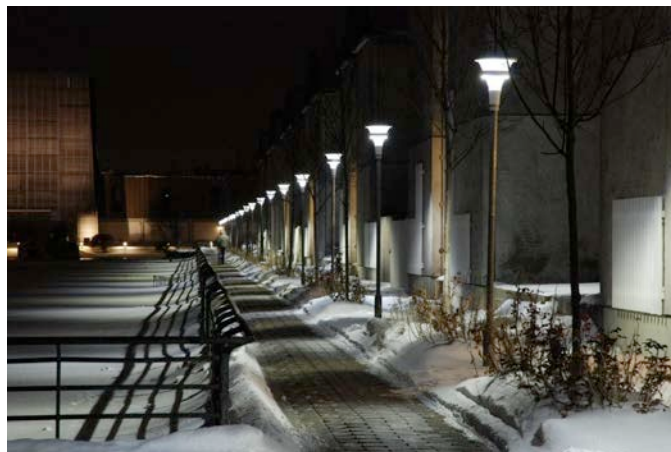
Figure 7: Albertslund street lighting (@ City of Albertslund)
